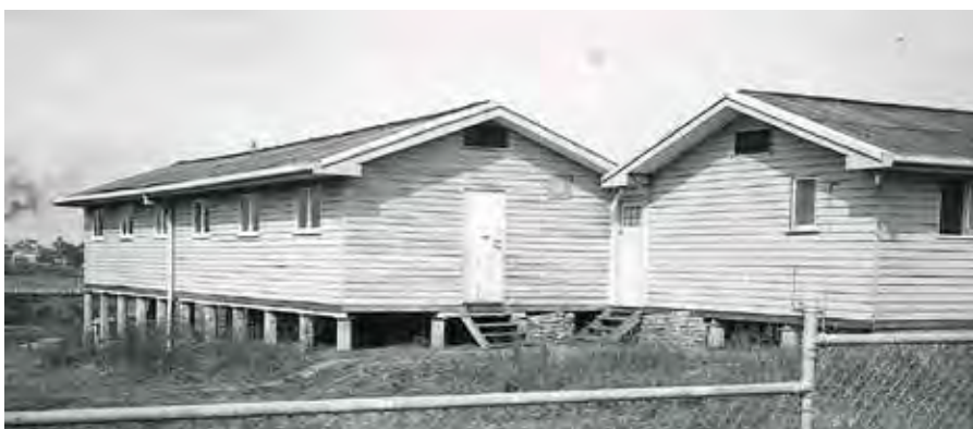
Above: South Street School site.
