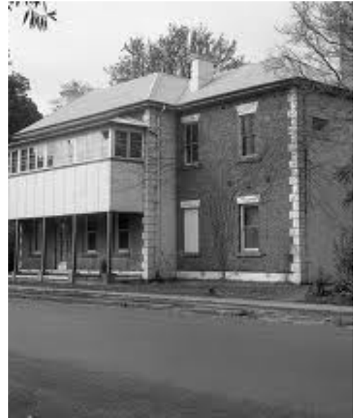
Above: Brough House, Church Street, Maitland, housed the first recorded meeting.
